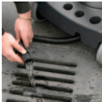
Drain hose system
